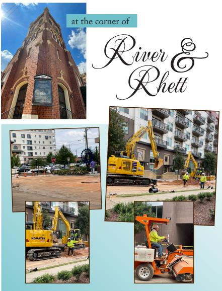
Beginning Monday, September 18, the City of Greenville began work on replacing the old, overloaded sewer main that runs along Rhett Street. Second Presbyterian Church ties into this sewer main that has needed replacement for many years as development is increasing in this area. The old sewer main is 50–100 years old. Rhett Street will be closed during the day until the work is completed in mid-October. ◆
